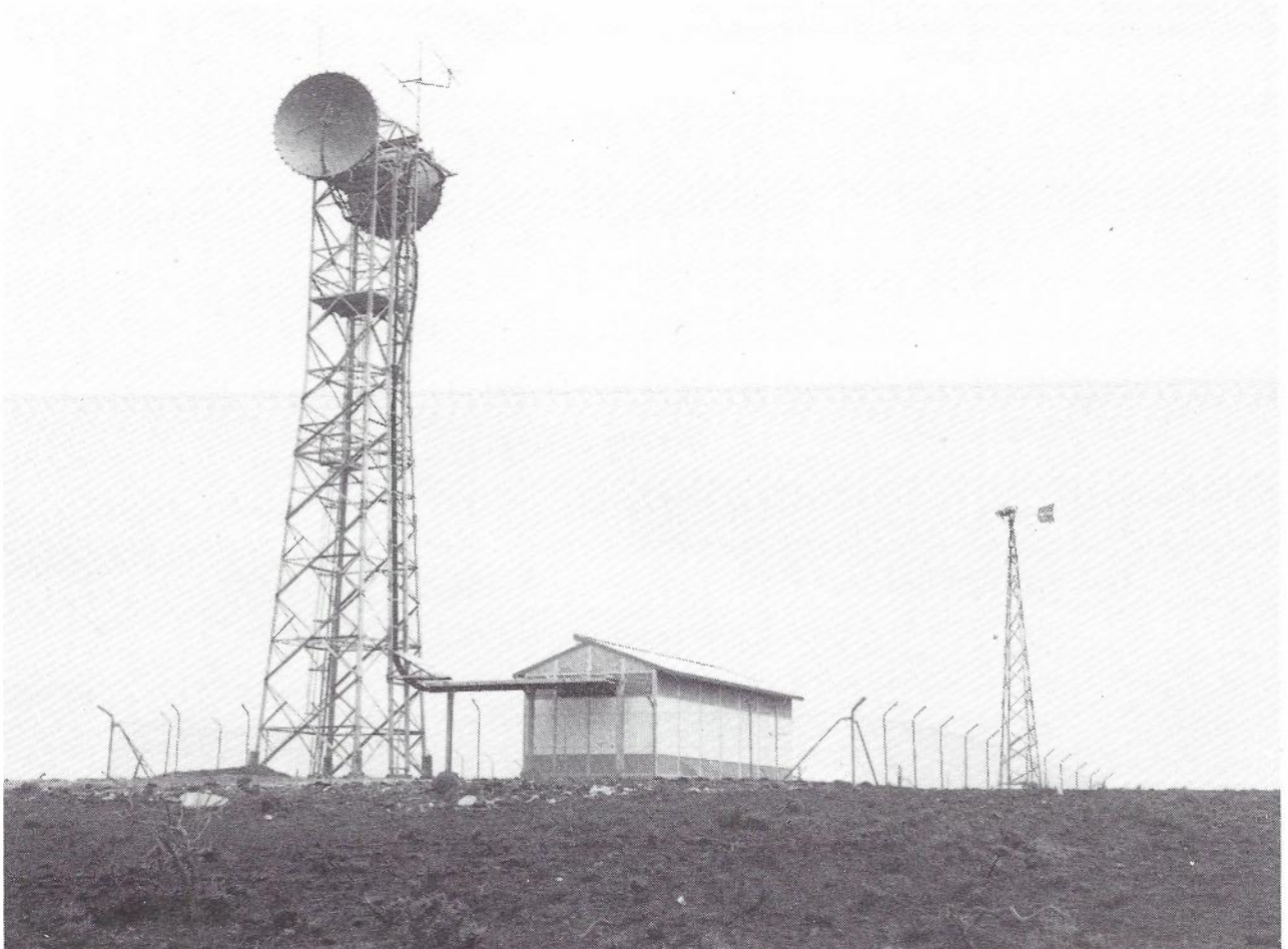
Fig. 5. A Repeater Station on the East-West Microwave Radio System.
