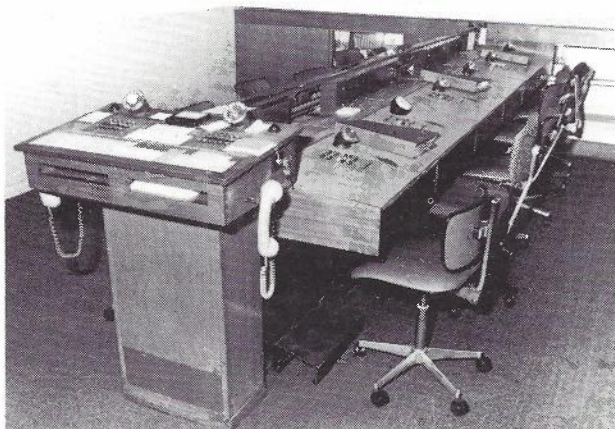
Fig. 3 — Typical pre SULTAN/LEOPARD Operator Positions.
