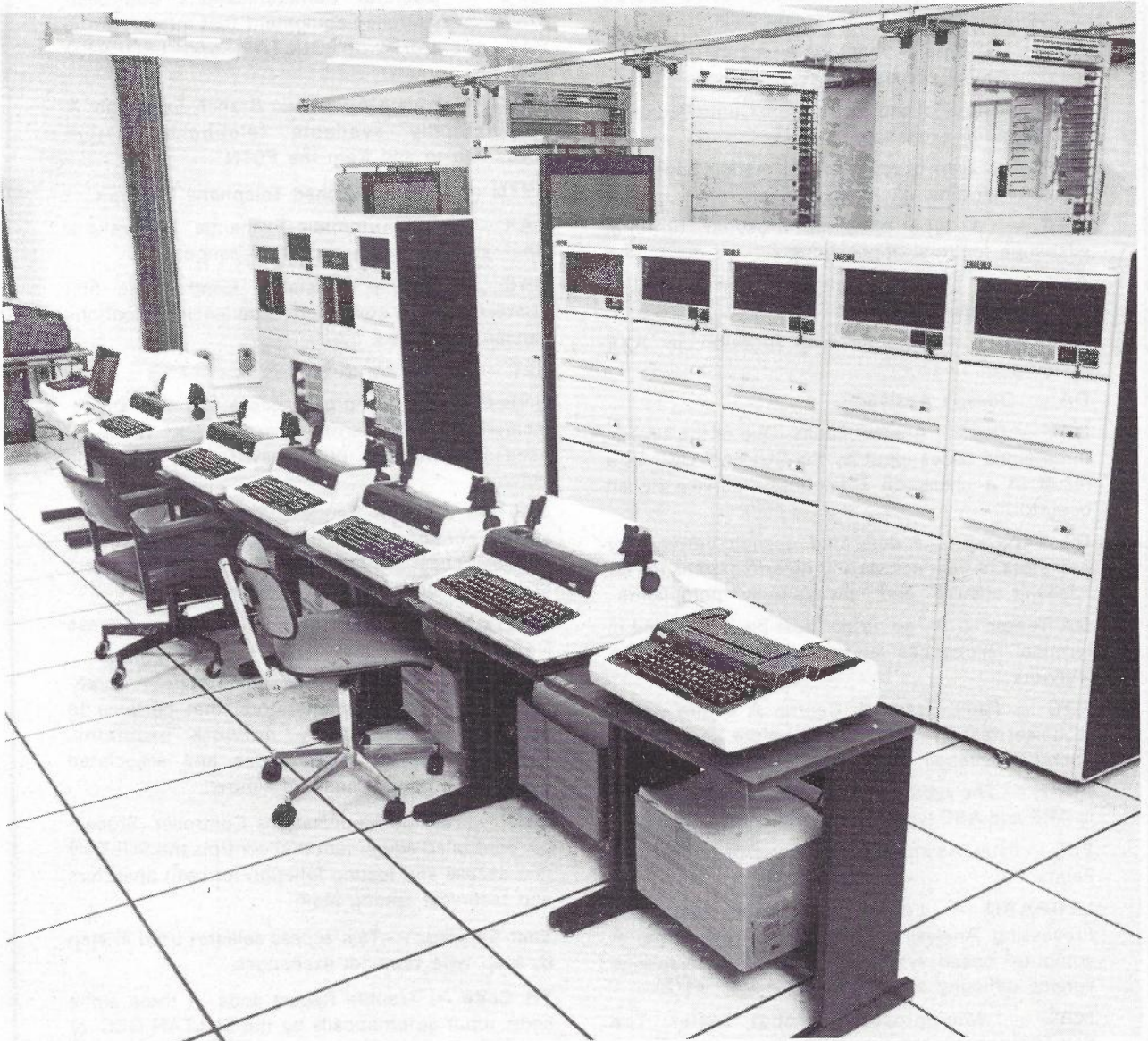
Fig. 15 — TCC and OCC Equipment at City East Building in Sydney, NSW. The system consoles are in front. Behind these are, from left to right, two OCCs, a modem cabinet and five TCCs. Associated crossbar type racks are to the rear, behind the minicomputer suite.
