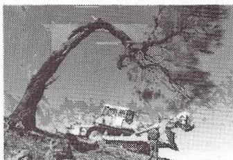
Cable Ploughing Tractor in action, ploughing in an optical fibre cable.
