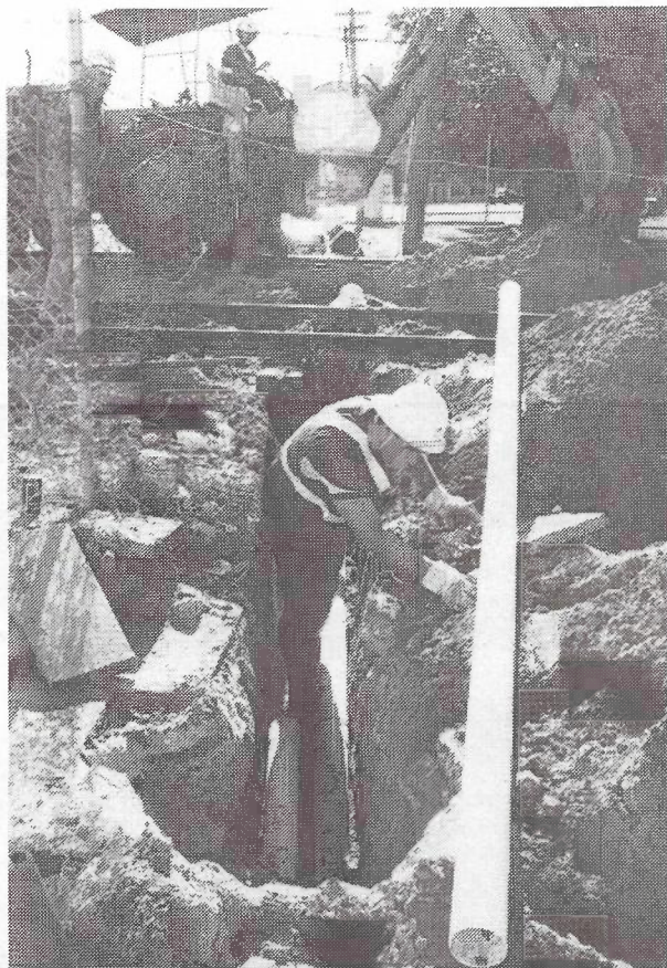
Ducting under the railway line in Fremantle, near Challenger Harbour.
