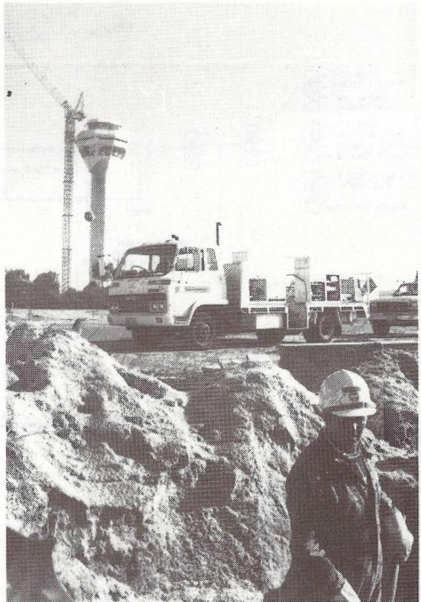
Conduit installation to the Qantas Facilities Building.
