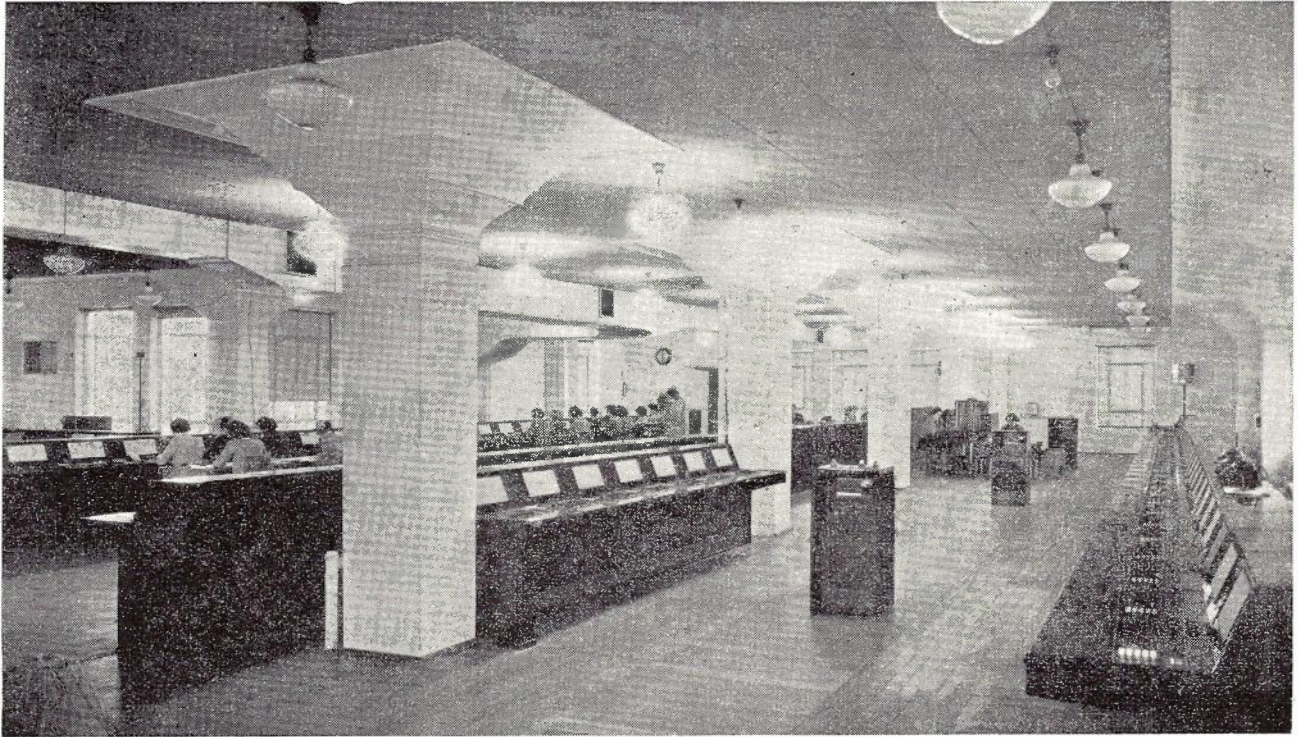
New Melbourne Trunk Exchange.
