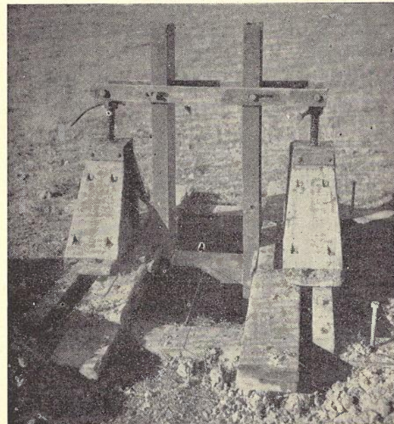
Fig. 2.—Channel Iron Footing for Poles.
