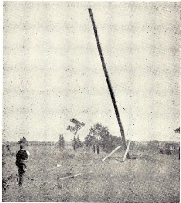
Fig. 8.—Sheer Legs Method—Final Stage of Erection.
