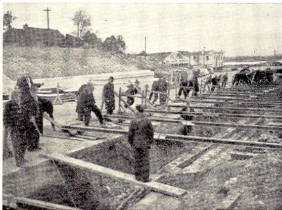
Fig. 3.—Ready for Rolling.
