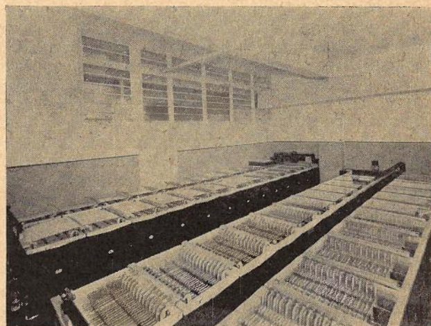
Fig. 1.—North Sydney Battery Room.
