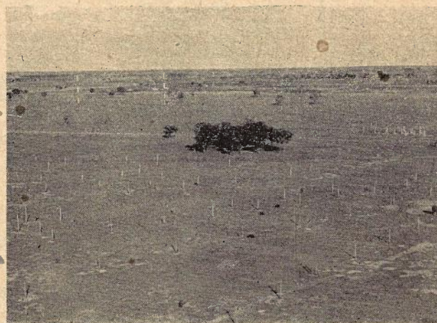
General view of site with masts and transmission lines.
