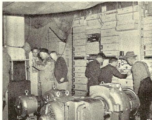
Fig. 5.—Restoration work in progress. (Reproduced by courtesy of "The Sydney Morning Herald.")
