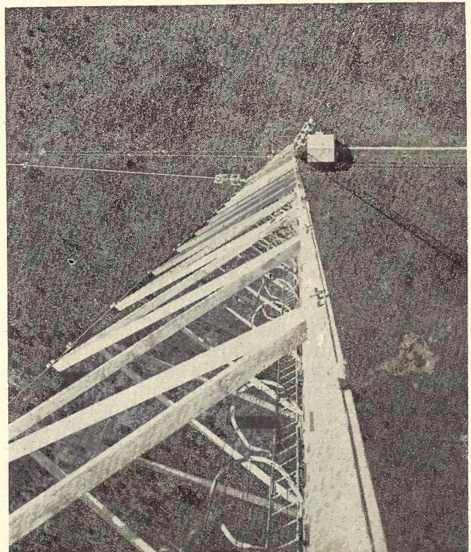
Fig. 6.—View looking down from the top platform of the 730 ft. vertical radiator used for 2FC and 2BL at Liverpool, N.S.W. Included in the photograph are portions of the bonding system, the protected internal ladder, and the guys, coupling hut and the coaxial transmission lines.
