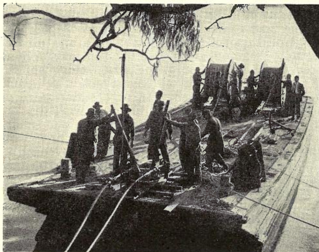
Fig. 5.—Barge at southern bank while cable being drawn ashore.
