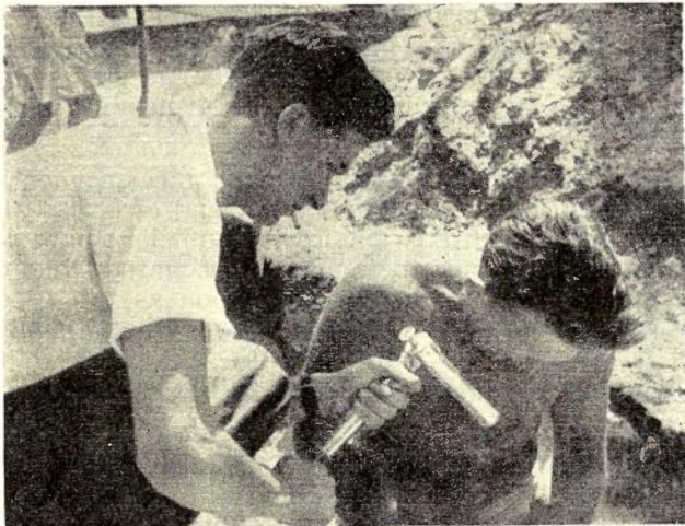
Fig. 6.—Dust sample being taken at manhole excavation, Bickle Road, Mosman, N.S.W.
