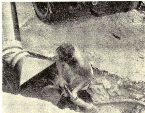
Fig. 8.—View showing Exhaust Unit working in open excavation.
