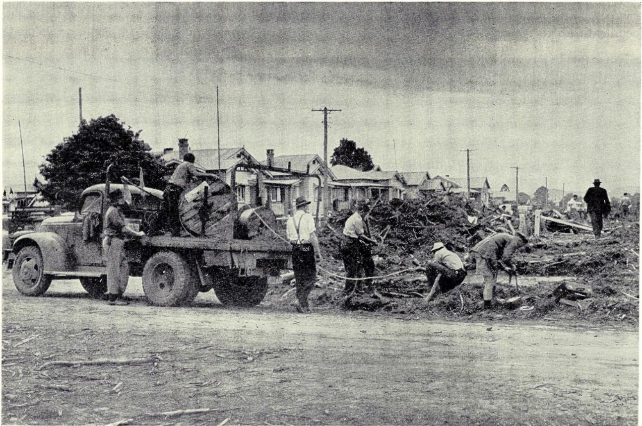
Fig. 5.—Kempsey Flood Scene.—Relaying cable amid debris piled shoulder high.
