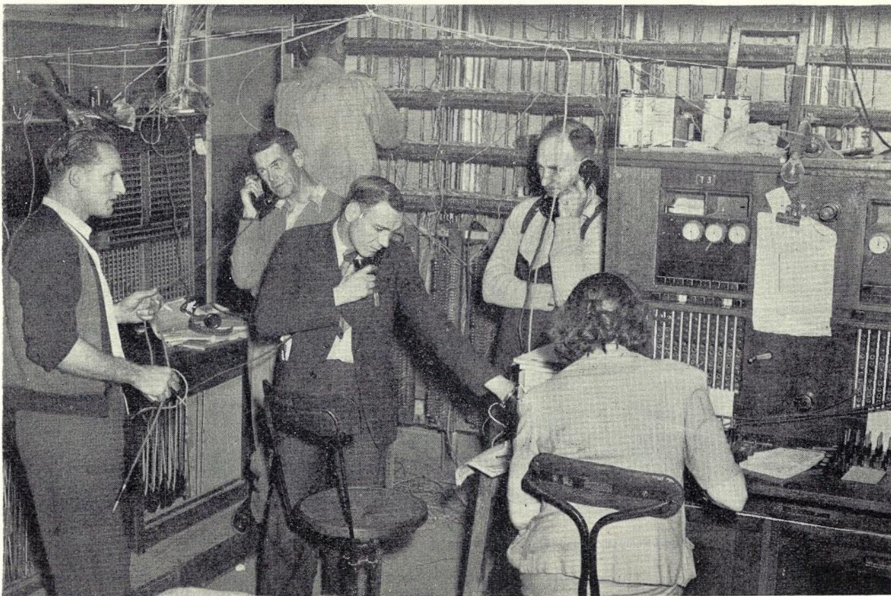
Fig. 4.—Checking Telephone Circuits, Kempsey. The camera records the detail of a flood-time emergency.
