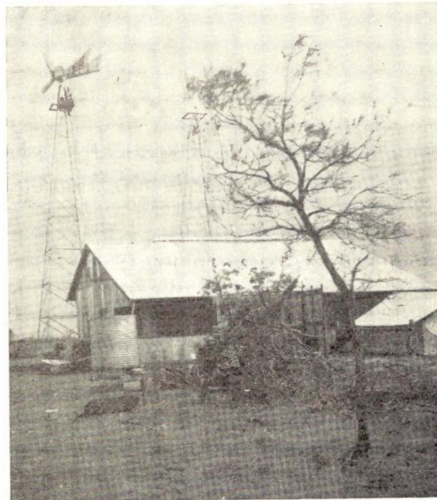
Fig. 17.—Sydney Williams "Steel Fram" Repeater Building.
