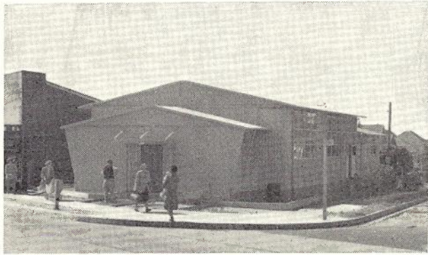
Fig. 25.—Post Office Building in Course of Erection
