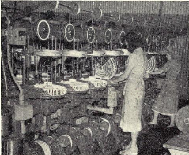
Fig. 3.—High speed paper insulating machine used for wrapping local type cables.
