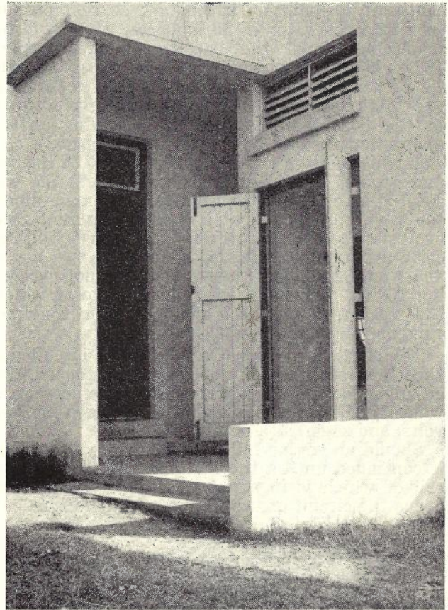
Fig. 24.—Entrance Lobby, showing Fixed Louvres.
