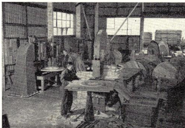
Fig. 13.—General view of drum making unit.
