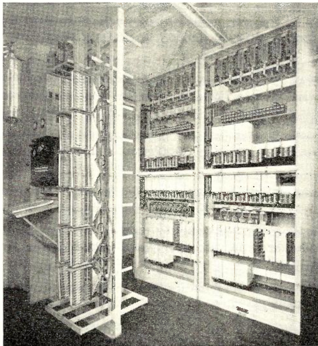
Fig. 11.—General view, showing equipment rectifier and batteries in the same room. Rectifier and battery cabinet at extreme left.
