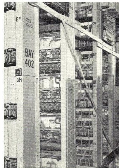
Fig. 3.—Working trunk boards braced to form solid block.
