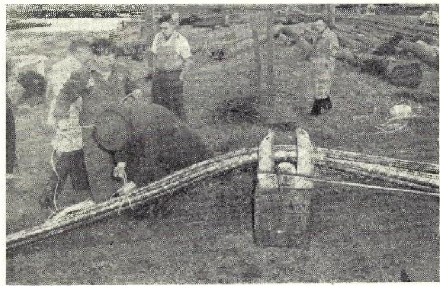
Fig. 8.—Cables being lashed together and passing over a guide roller.
