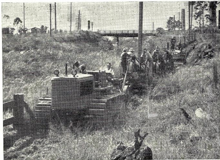
Fig. 3.—Mole plough in operation.
