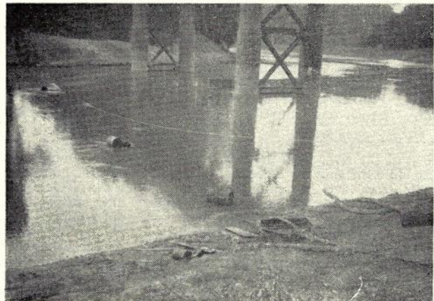
Fig. 4.—General view of crossing, showing drag scraper bucket and drums used to float cable.
