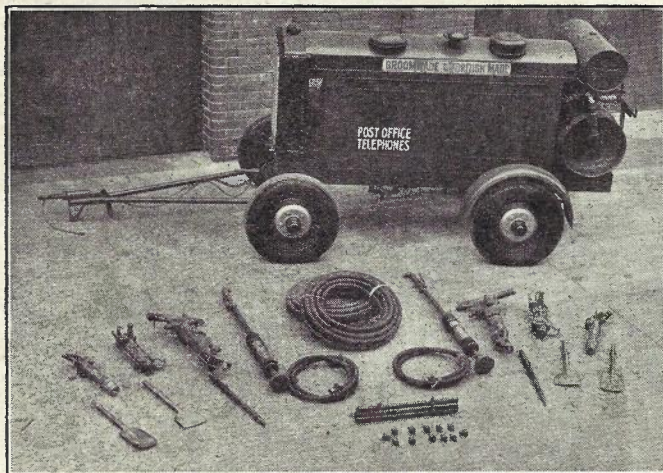
FIG. 4.—TWO-TOOL TRAILER AIR-COMPRESSOR AND TOOL EQUIPMENT.
