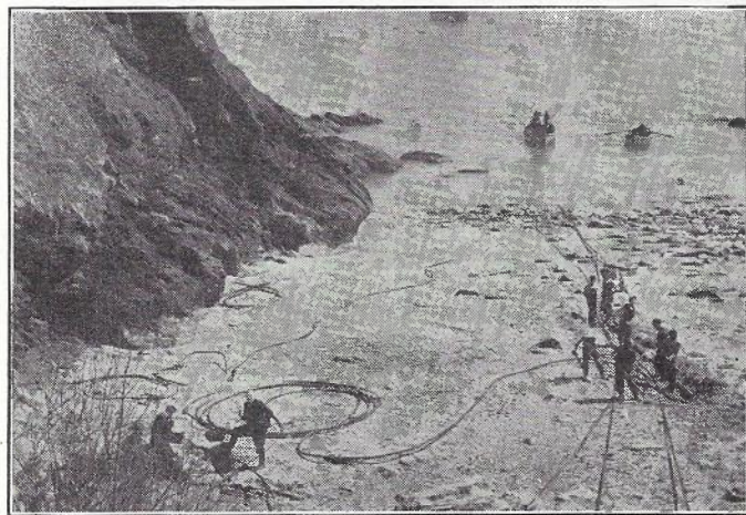
TESTING ONE OF THE SHORE ENDS.
