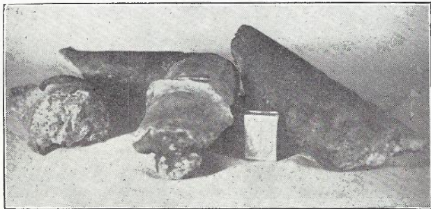
FUNGUS FORMATION REMOVED FROM DUCT.
