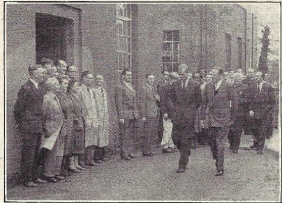
RETURNING FROM NEW WORKSHOP BUILDING.
