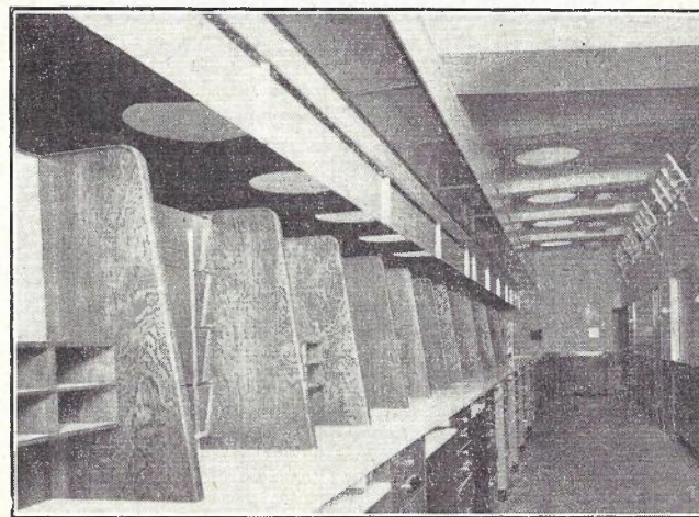
THE COUNTER LIGHTING INSTALLATION.
