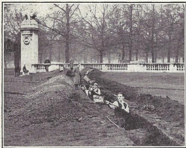
FIG. 2.—EXCAVATING FOR DUCT ROUTE NEAR CANADA GATE.
