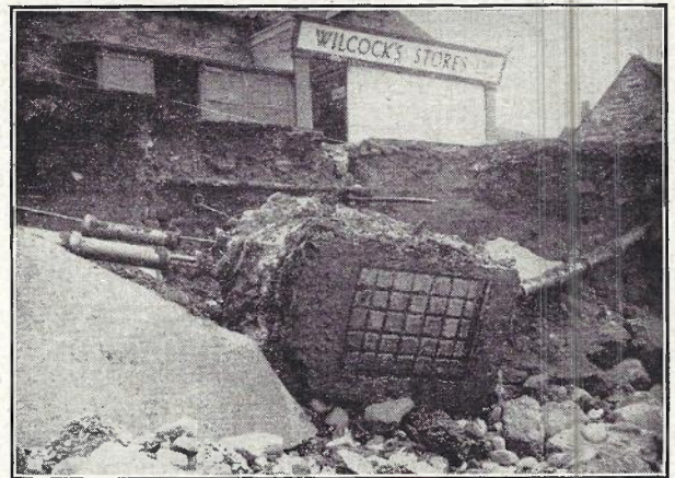
THE JOINT BOX SUSPENDED ON CABLES.
